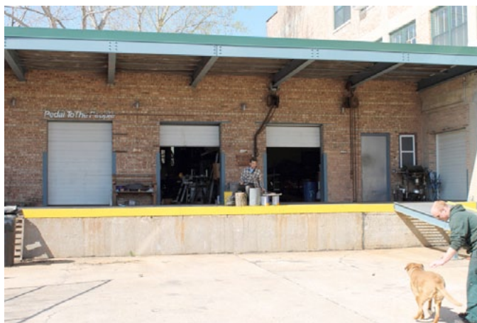
The loading area of the building.
